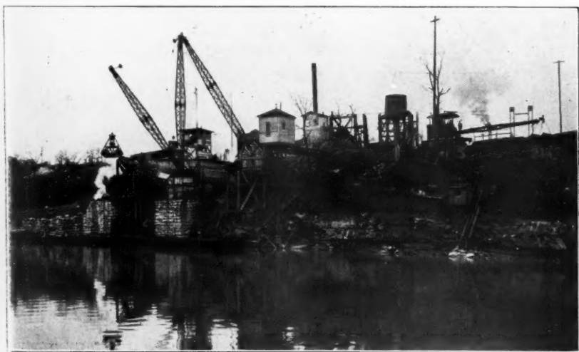
Unloading Kyrock from Barges.
